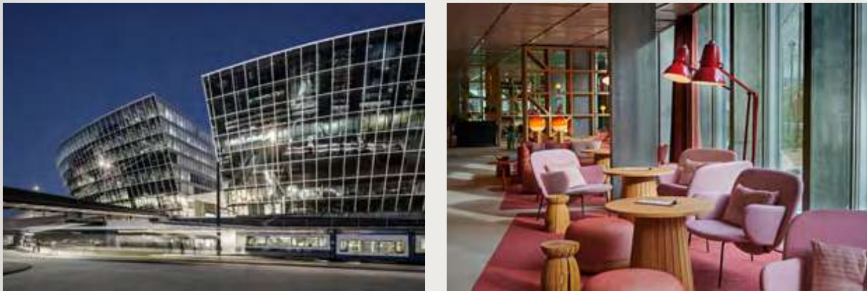
HYATT PLACE ZURICH AIRPORT THE CIRCLE ZURICH
